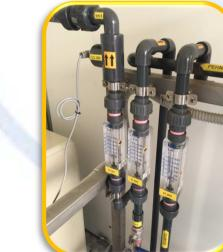
From the membranes comes the PERMEATO, pure water, a CONCENTRATED WASTE and a RICYCLE The flow rate of these is measured by flow meters The total production of pure water is the sum of the recirculation plus the permeate
