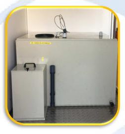
The osmotic water (PERMEATO) is sent to the storage tank in polypropylene and anti-lapping with level sensors to detect high / low level alarms or lack of osmotic water
