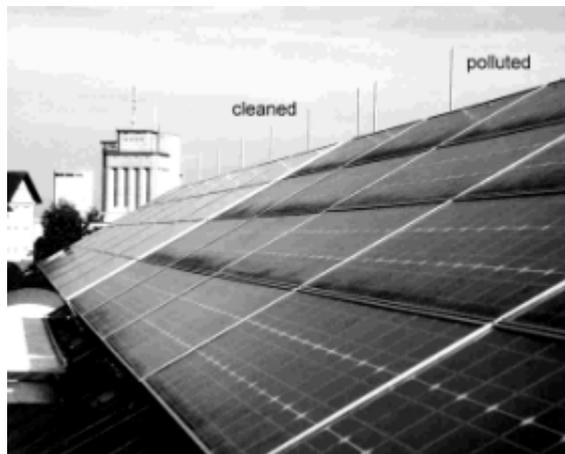
**Fig. 2:** View of a part of the PV array with visible pollution. The modules at the left side are cleaned, whereas the others show the pollution accumulated from summer 1993 to fall 1997.
