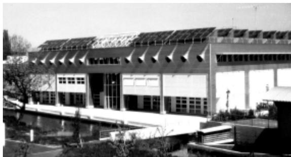
**Fig. 1:** View of the building of the department of Electrical Engineering of HTA Burgdorf with a PV generator of 60kWp on top of the roof.
