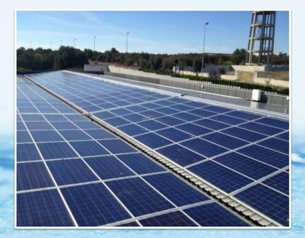
On the surface of these panels on the roof of a manufacturer of animal feed can be noticed residues of pork rinds, together with droppings of seagulls. The residues deposited on the panel and, mainly due to the heat, became scaled very difficult to remove.
